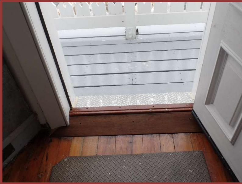
Completed exterior threshold
