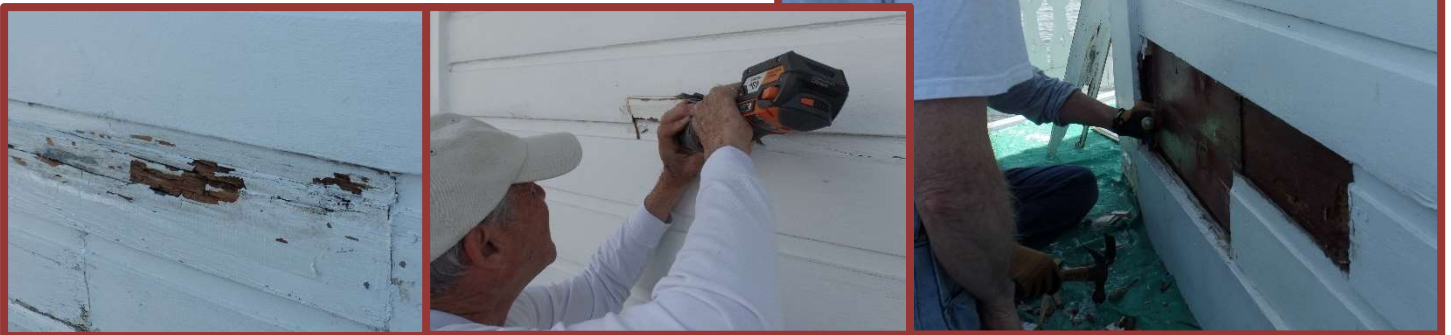
Rotted siding – original condition and repairs in progress
