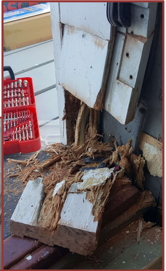
View of the extent of the rotted threshold
